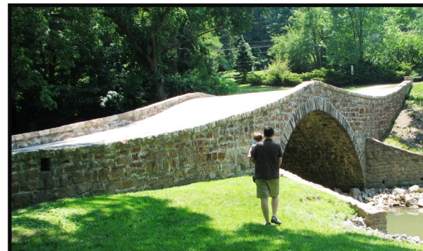
Stone Arch Bridge
